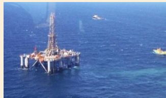
Upstream Project Kudu Offshore Gas field
